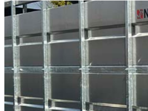
Incorporated box section for strength and reinforcement.
