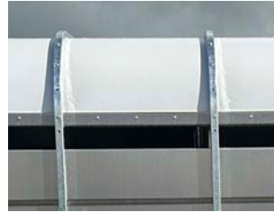
Aluminium spouting reinforces the roof.
